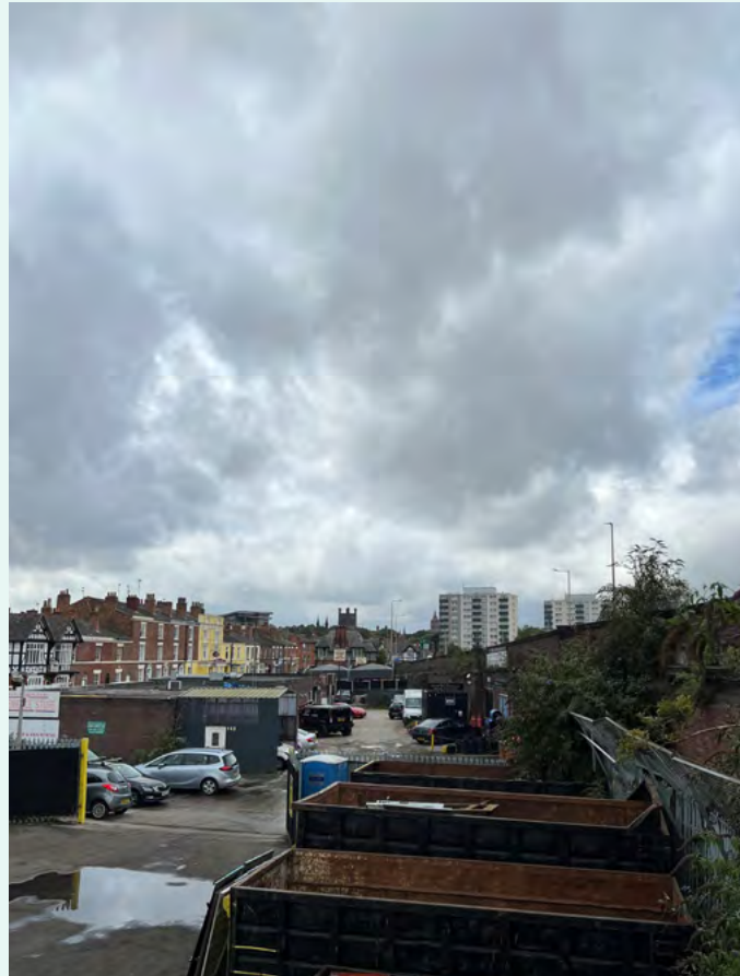
Hoole Bridge access staircase to Brook Street north
